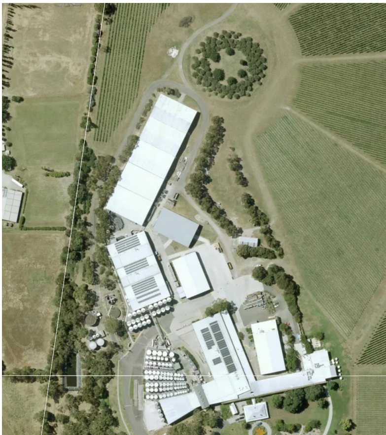
Figure 2 - Aerial Photo development area (January 2022)
